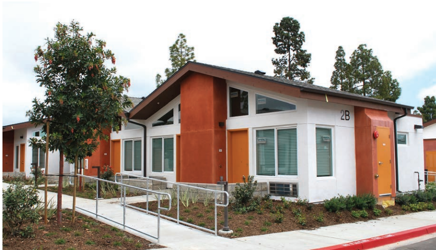
Vista Series 4000 windows installed at Levant Senior Cottages. Photo courtesy of Crystal Pacific Window & Door Systems.
